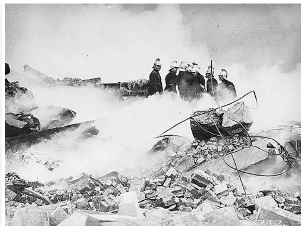
Firemen on the site of Goldsbrough Mort's wool store, Pyrmont, Sydney, September 26, 1935. The fire which destroyed the six story wool store at Pyrmont was the worst in Sydney since 1921. 230 firemen worked to stop it spreading to nearby buildings. 20,000 bales of wool were lost. PHOTO: STATE LIBRARY OF NSW
